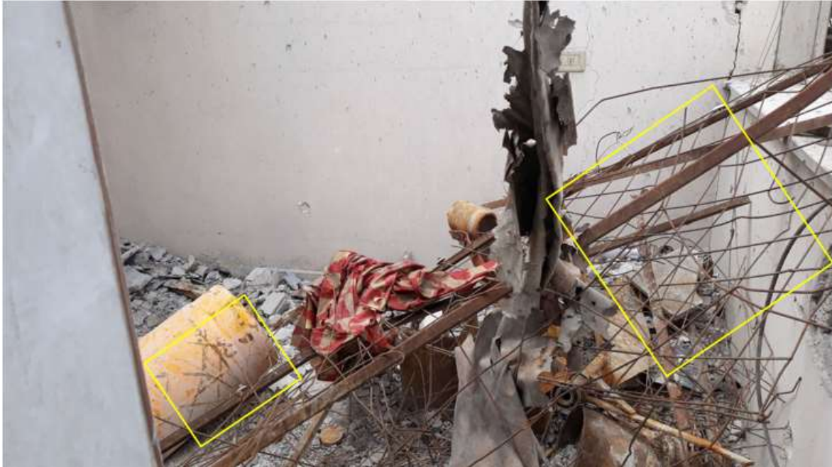
FIGURE 12: VISIBLE SQUARE-PATTERNED DAMAGE ON THE CYLINDER'S BODY RESEMBLING THE GRID PATTERN OF THE METAL MESH LOCATED ON THE ROOFTOP. (SOURCE: FFM)
