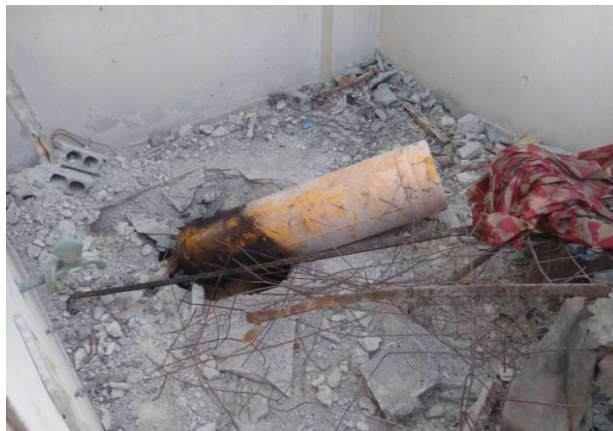
FIGURE 29: THE CYLINDER ON THE BALCONY AT LOCATION 2, SHOWING A GRID PATTERN CORRESPONDING TO THE METAL MESH
