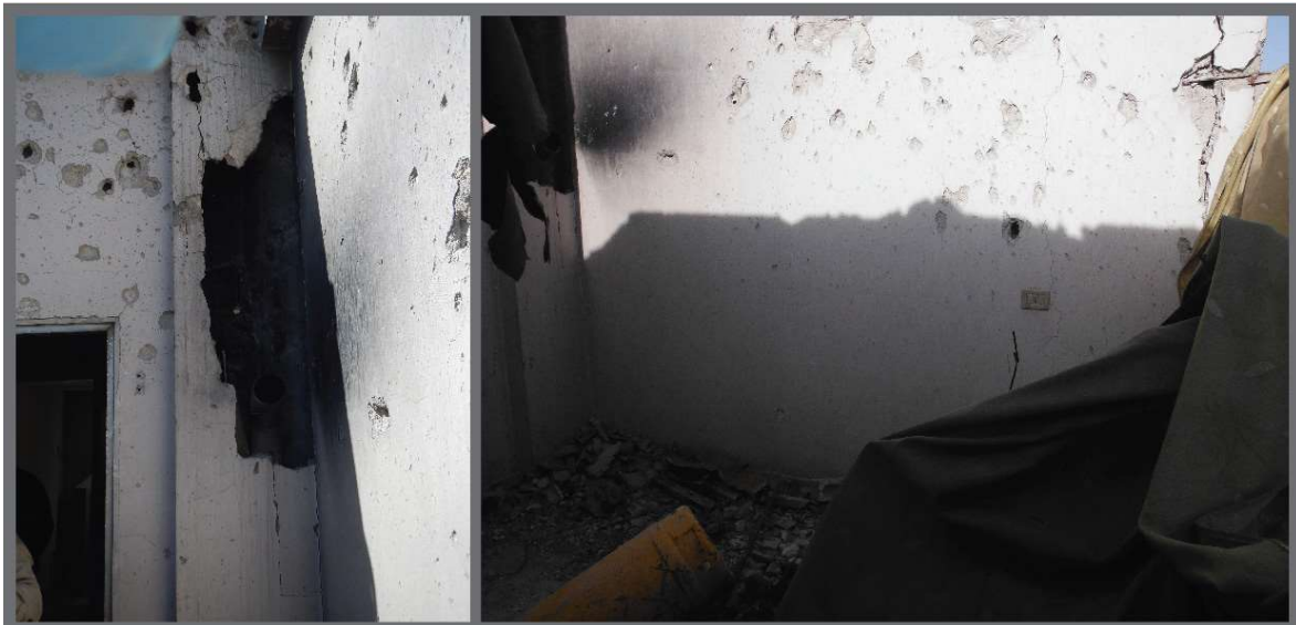
FIGURE 18: PHOTOS OF THE UPPER PART OF THE ROOFTOP WALLS. THE FRAGMENTATION PATTERN IS NOT CONSISTENT WITH AN EXPLOSIVE EVENT (SOURCE: FFM)
