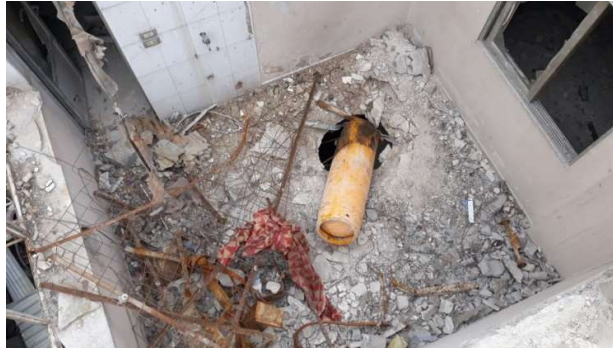
FIGURE 28: CYLINDER ON THE ROOFTOP FLOOR AT LOCATION 2
