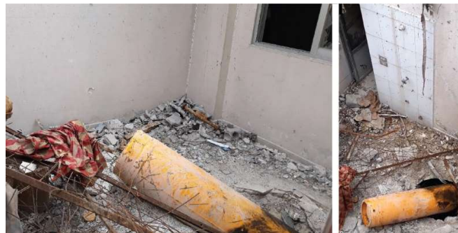
FIGURE 52: NARROW DOOR AND WINDOW'S OPENING (SOURCE: FFM)
