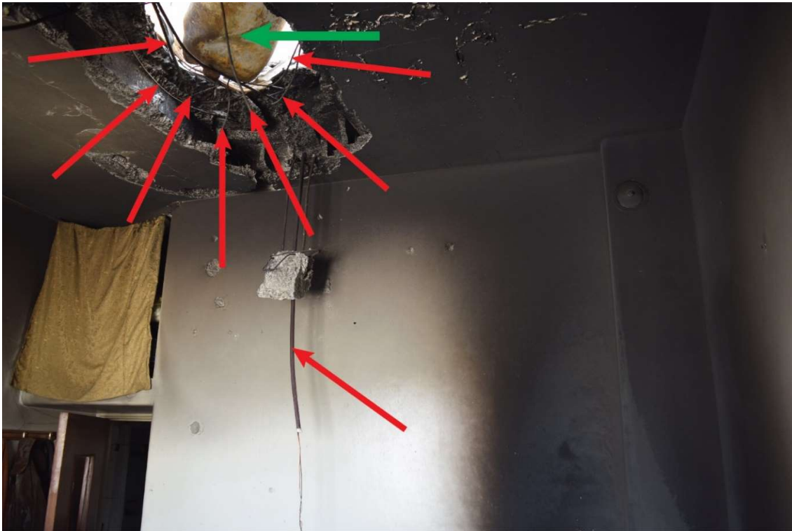
FIGURE 37: VISIBLE DEFORMATION OF THE STEEL REBARS IN THE CONCRETE TOWARDS THE INTERIOR OF THE BUILDING AT LOCATION 2.
