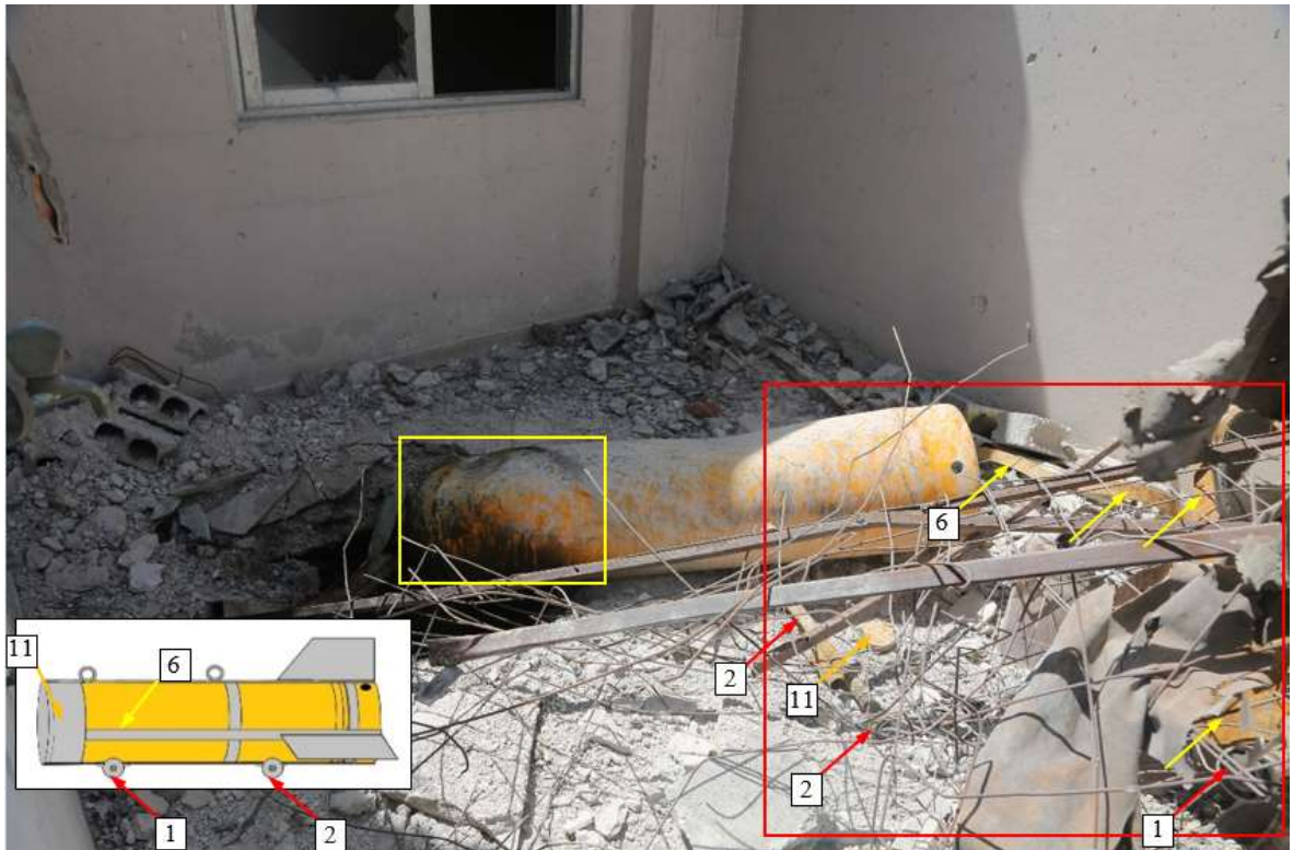
FIGURE 19: VISIBLE IMPACT CRATER, YELLOW INDUSTRIAL CYLINDER AND THE REMAINS OF THE METAL CRADLE, PARTLY TANGLED IN THE METAL MESH ON THE ROOFTOP.
